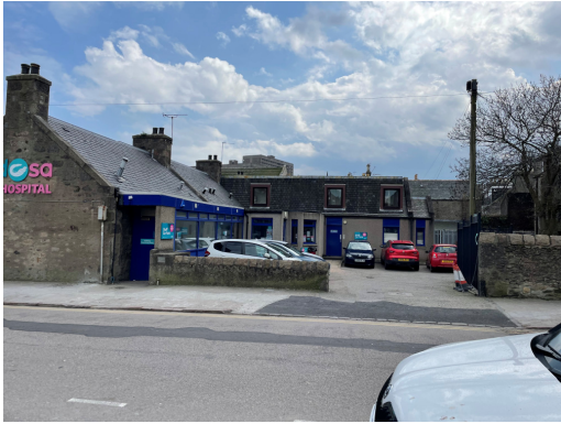
c) Two storey building to the North East, 26-30 Fraser Place with a mixture of materials.
