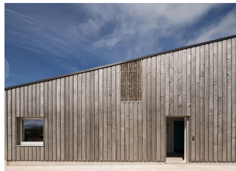
b) Scotlarch cladding.
