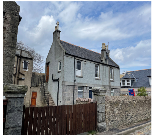
b) Two storey building immediately to South West, 5-7 Charles Street. Granite lower walls and harling above. Similarities to appeal site with varying lower & upper wall finishes.
