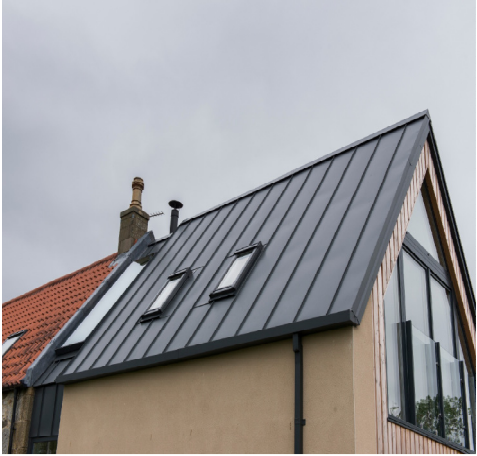
c) Grey standing seam metal cladding.
