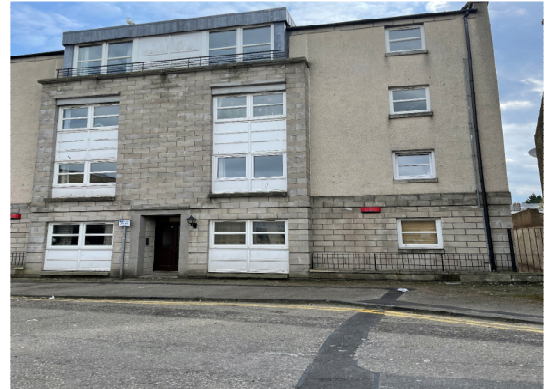
d) Four storey building to South East on Charles Street.
